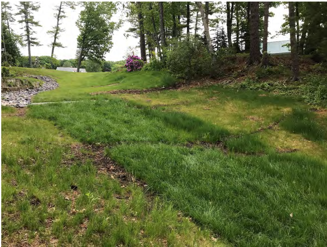
Fig 10: Slope below the manhole at Gundalow Landing/east side of the bay. Viewing east. (06-01-21)
