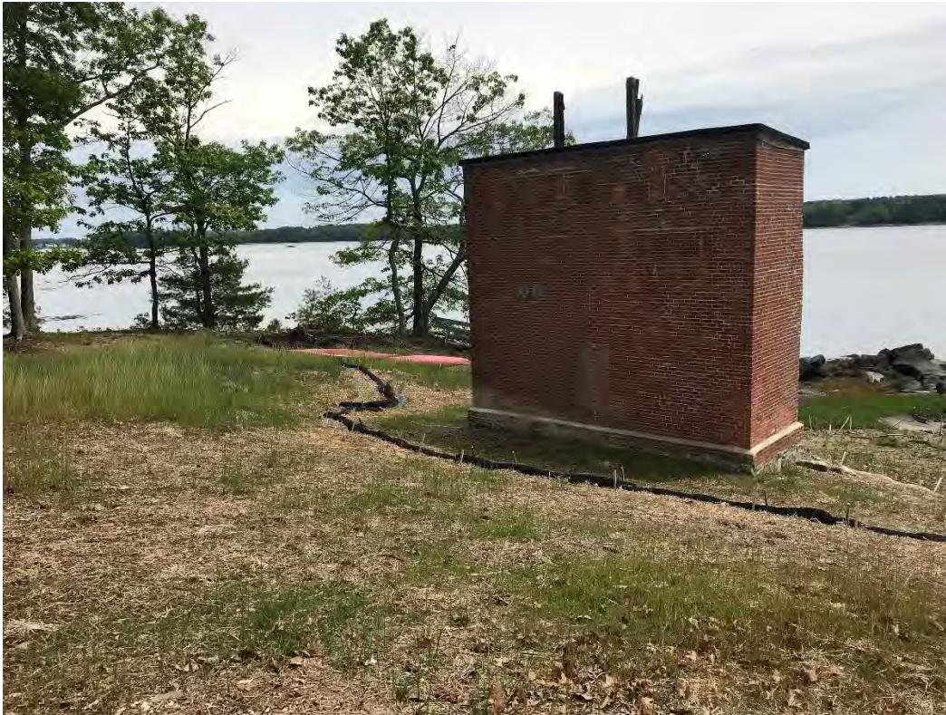
Fig 1: Slope leading down to cable house and salt marsh restoration at the west side of the bay. Viewing northeast. (06-01-21)
