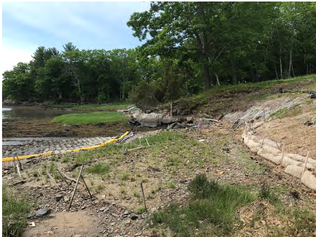
Fig 4: Toe of the slope and salt marsh restoration at the west side of the bay. Viewing south. (06-01-21)
