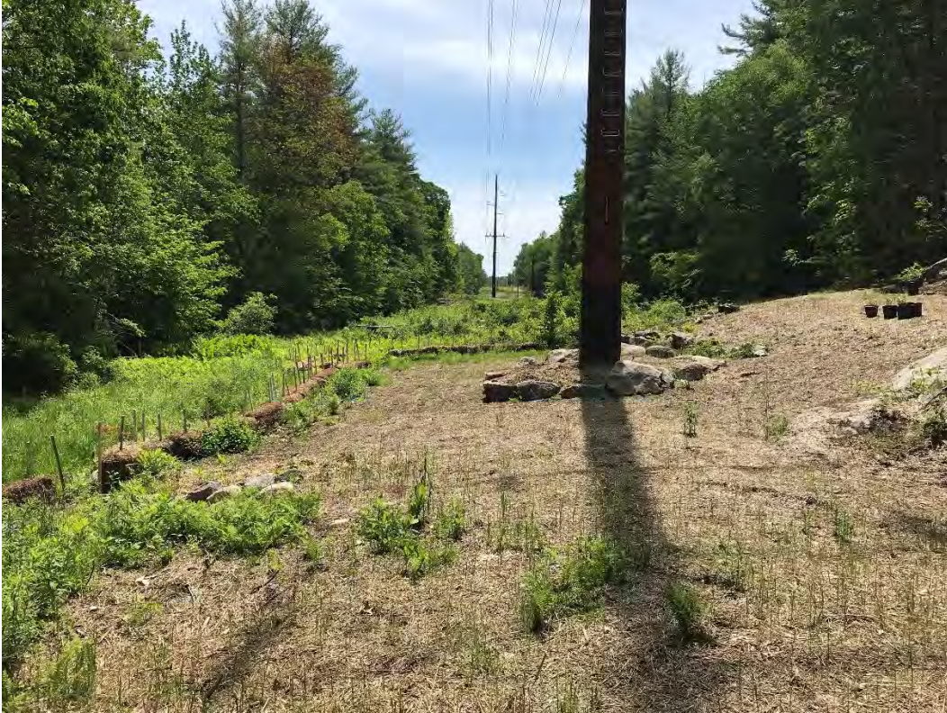
Fig 5: Str. 89 work area. Viewing southeast. (06-01-21)
