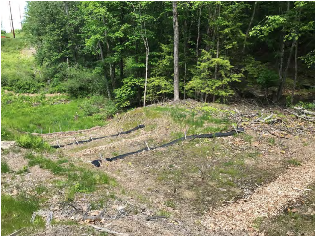
Fig 8: Lower portion of slope between Strs. 28 and 29. Viewing northeast. (06-01-21)
