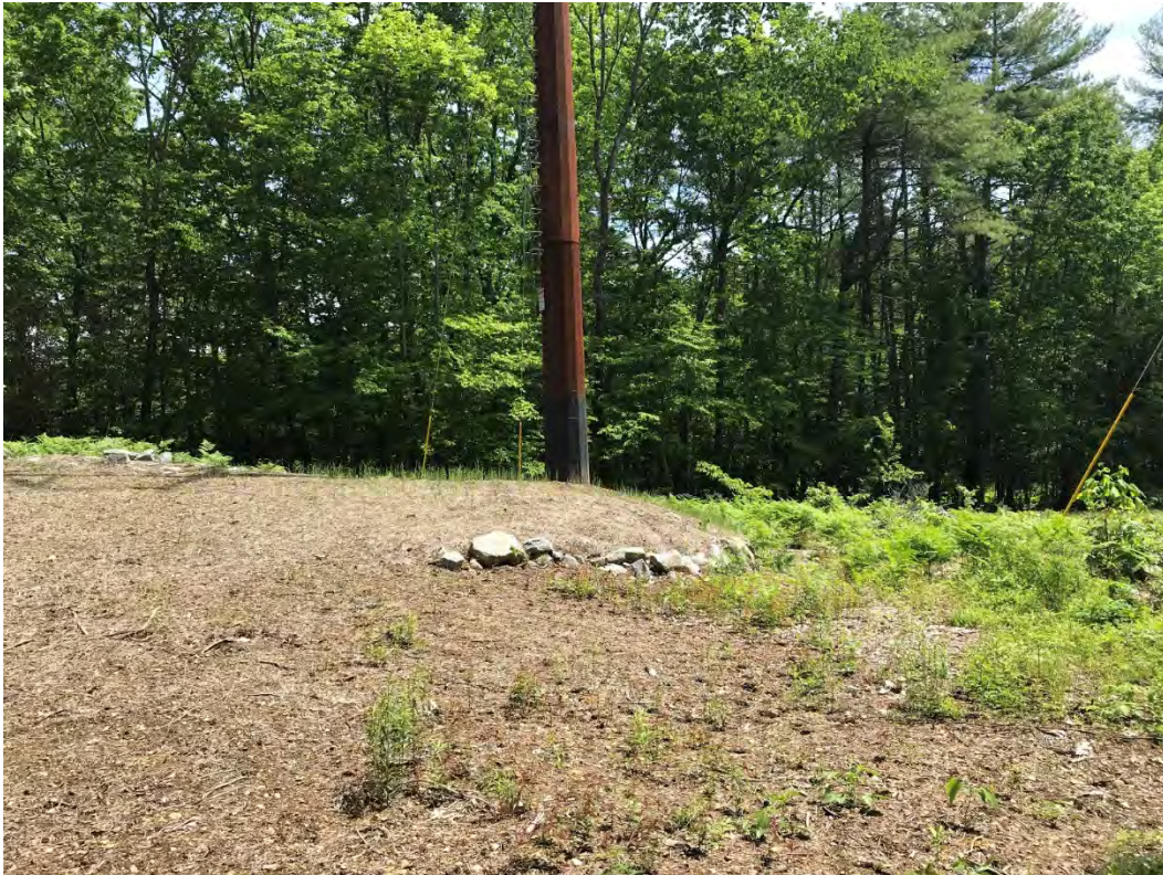
Fig 6: Str. 90 work area. Viewing northeast. (06-01-21)
